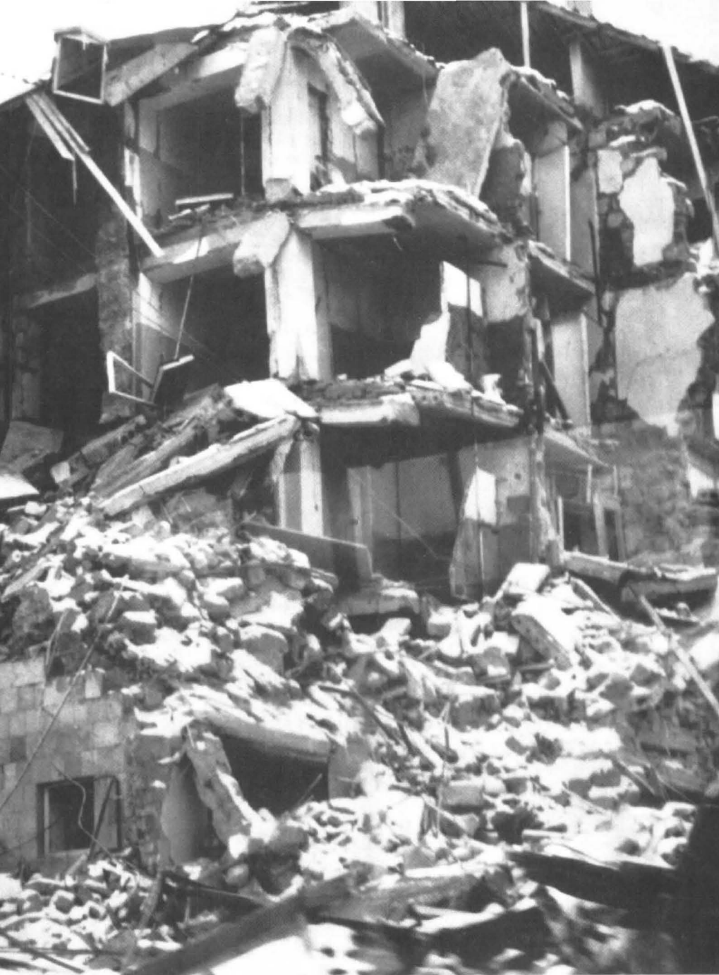
Apartment house in Spitak, Armenian Republic, destroyed by an earthquake in December 1988 that registered 6.9 on the Richter scale. Such apartment houses were not designed, or built, to withstand seismic activity of that magnitude. The earthquake claimed 25,000 victims. Courtesy United States Geological Survey
